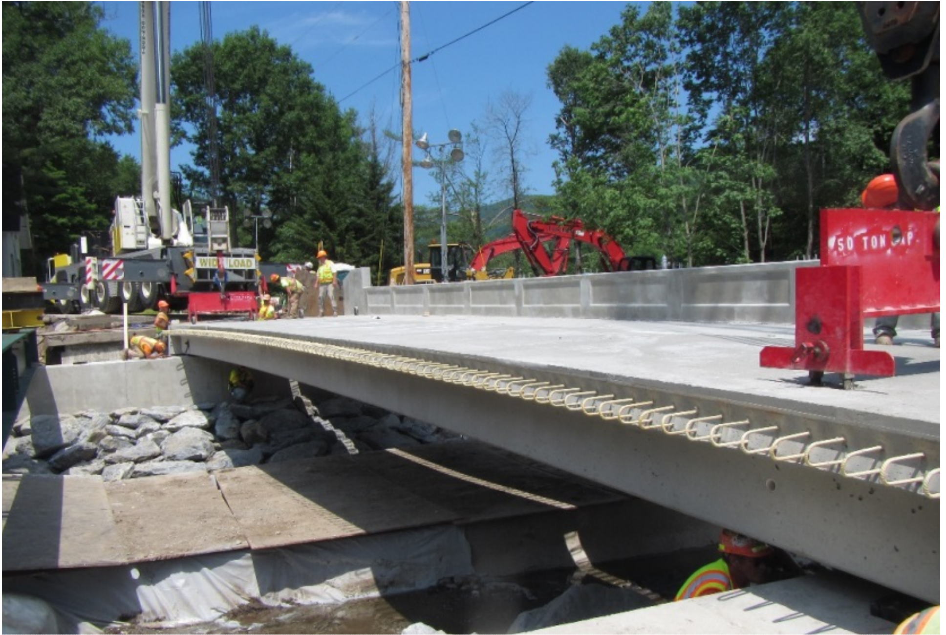
Superstructure – Precast Pre-stressed Concrete NEXT Beam Bridge
