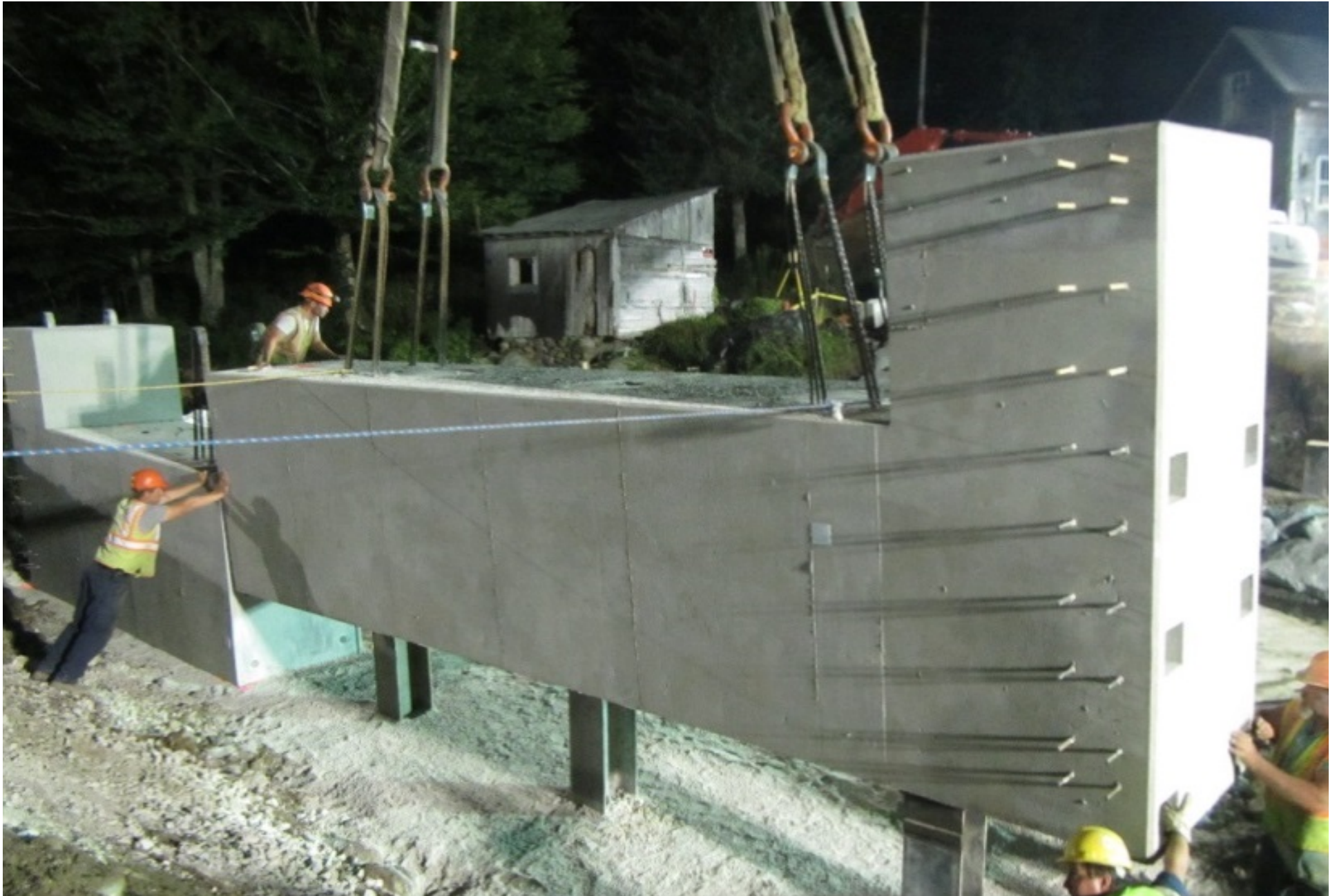
Substructure – Precast Concrete Integral Abutment on Steel Piles
